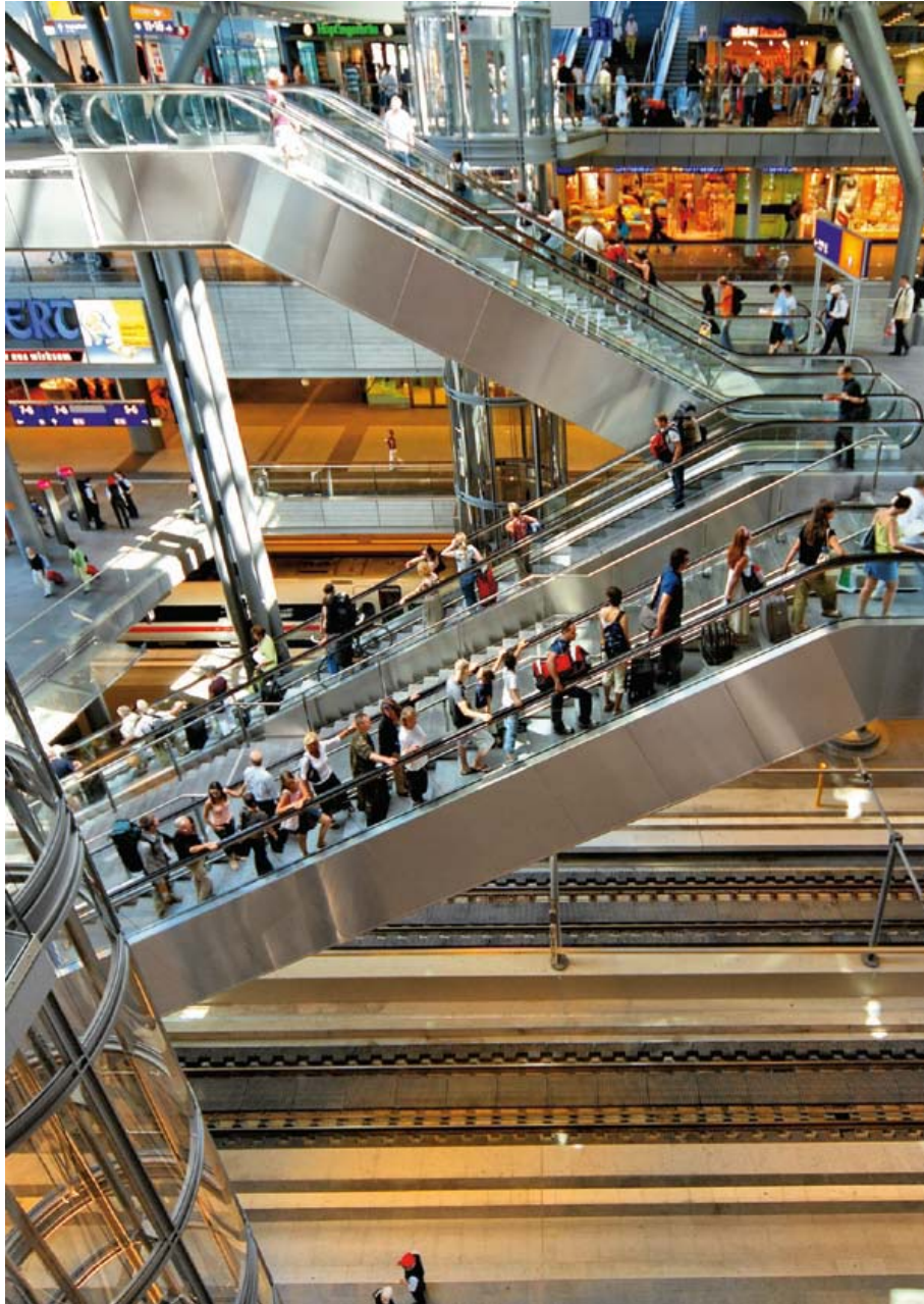
Photograph 3 — Escalator handrail height (Courtesy KONE™)
